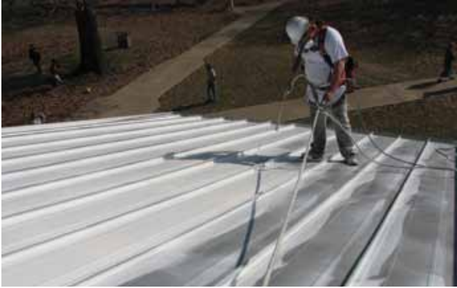
ABOVE ▲ The Coraflon product has a 16.2 to 1 ratio, making it more complicated to apply than coatings that have a 1:1, 2:1, or even 3:1 ratio. “There is a definite learning curve when applying the product,” relates Ruff.
